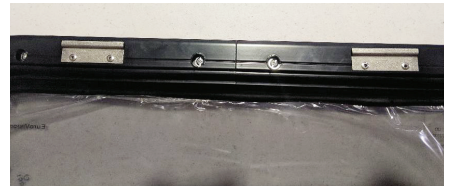
Stainless Steel lugs holding the blind assembly to the window.
